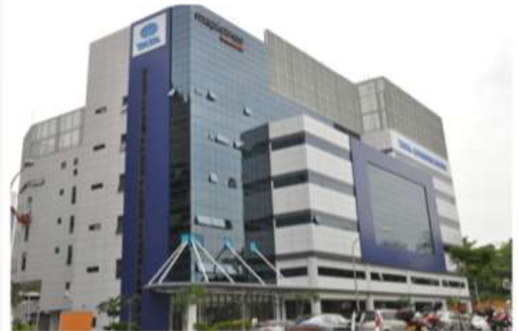
Example of BTS – Tata Communications Exchange
