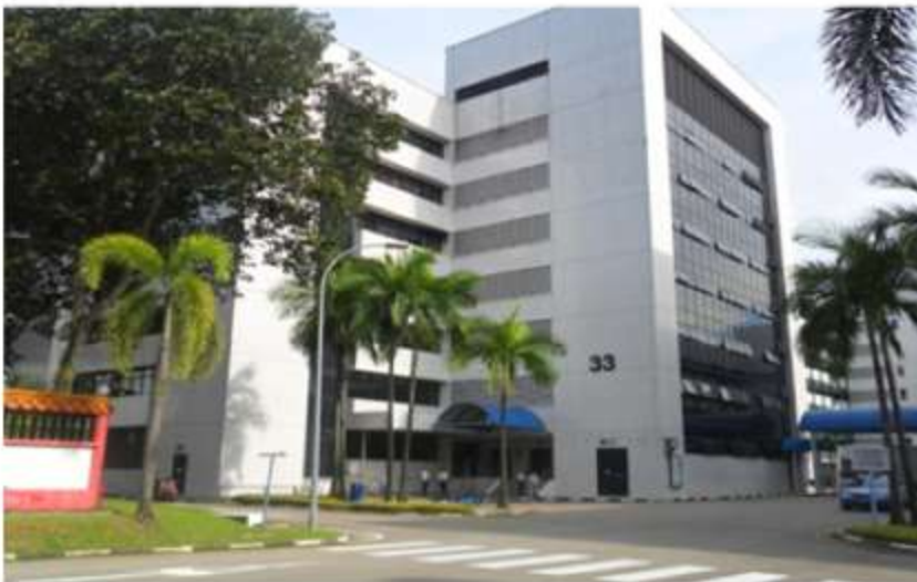
Woodlands Central Cluster before redevelopment
