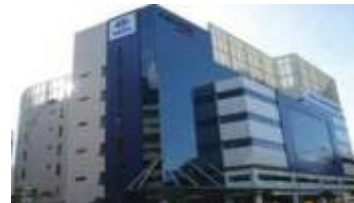
● Tata Communications Exchange
